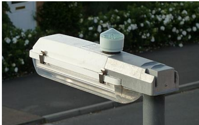
Figure 1: Street Lamps with Light detectors on top of it (Source: http://www.bradleystokejournal.co.uk/ )
